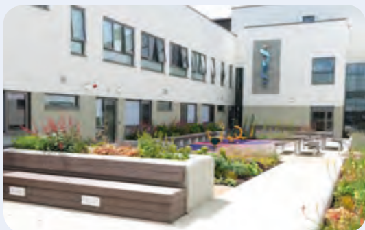
Boyle Primary Care Centre
