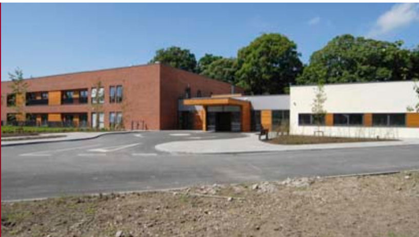
New 50 bed Community Nursing Unit at St. Mary's Orthopaedic Hospital, Cork.
