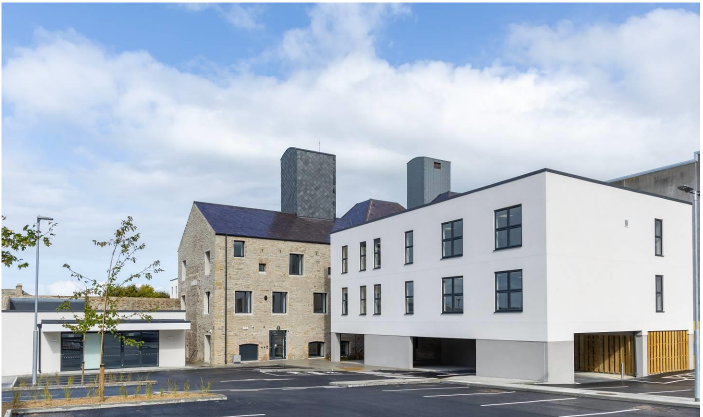
Roscrea Primary Care Centre, Co. Tipperary
