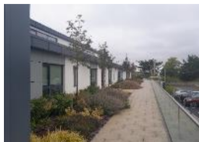
Kanturk Community Nursing Unit
