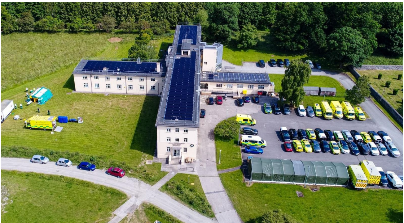
Solar Panel Installation Project, HSE National Ambulance Training Centre, Phoenix Park, Co. Dublin
