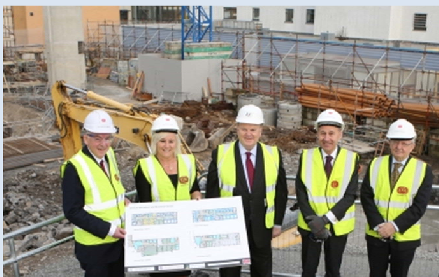
Inspecting building works at the Clinical Education and Research Centre, University Hospital Limerick were (L-R): Prof. Don Barry, President, University of Limerick; Prof. Colette Cowan, CEO, UL Hospitals; Minister for Finance, Michael Noonan TD; Prof. Michael Larvin, Head of UL's Graduate Entry Medical School; and Prof. Niall O'Higgins, Chairman, UL Hospitals
