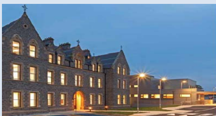
Ballyshannon Primary Care Centre
