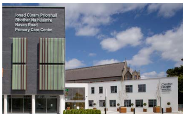
Navan Road Primary Care Centre (Photo: Paul Tierney)
